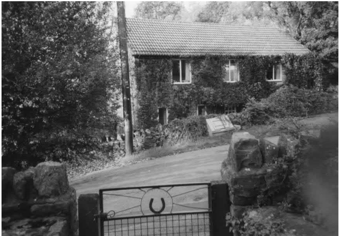
House built on site of the Mill Pond and Race (2005 P. Alcock)
