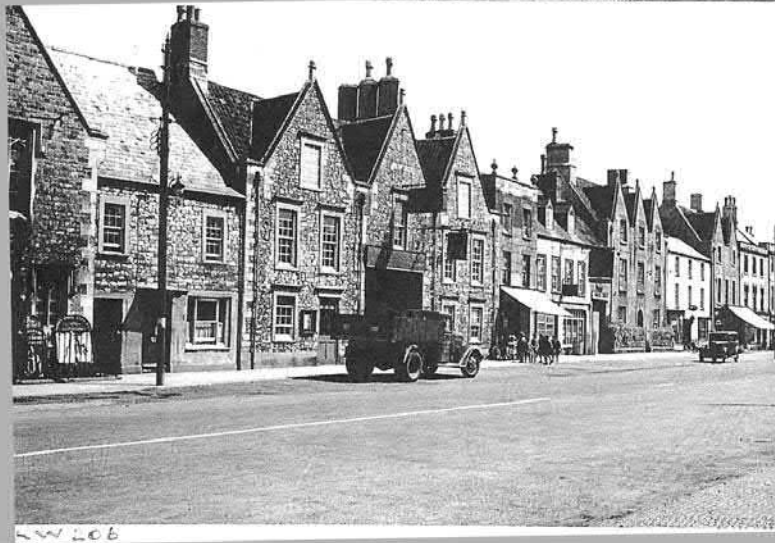
Broad Street Scene with The George Hotel in Centre.
